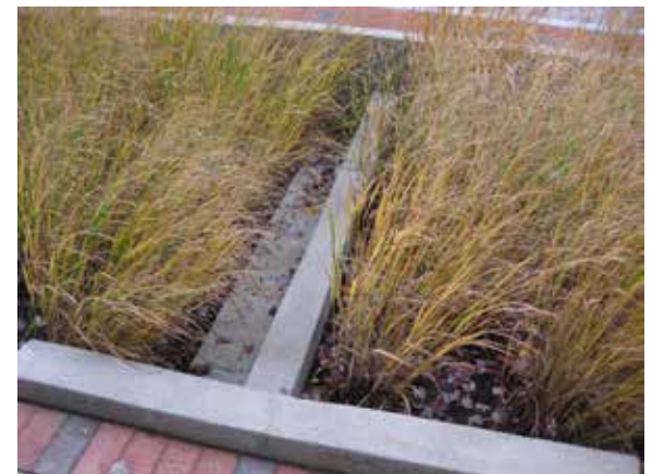
A check dam inside a tree box bioretention planter slows down the flow of water and encourages infiltration.
