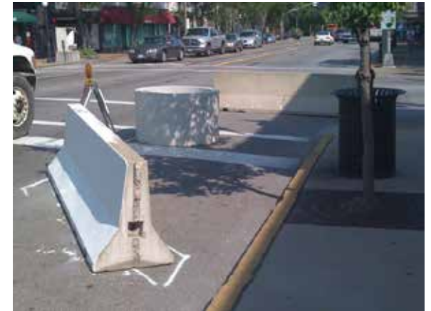
Figure 11-1 Temporary Curb Extensions in South Grand Road Diet Project, St. Louis, MO
