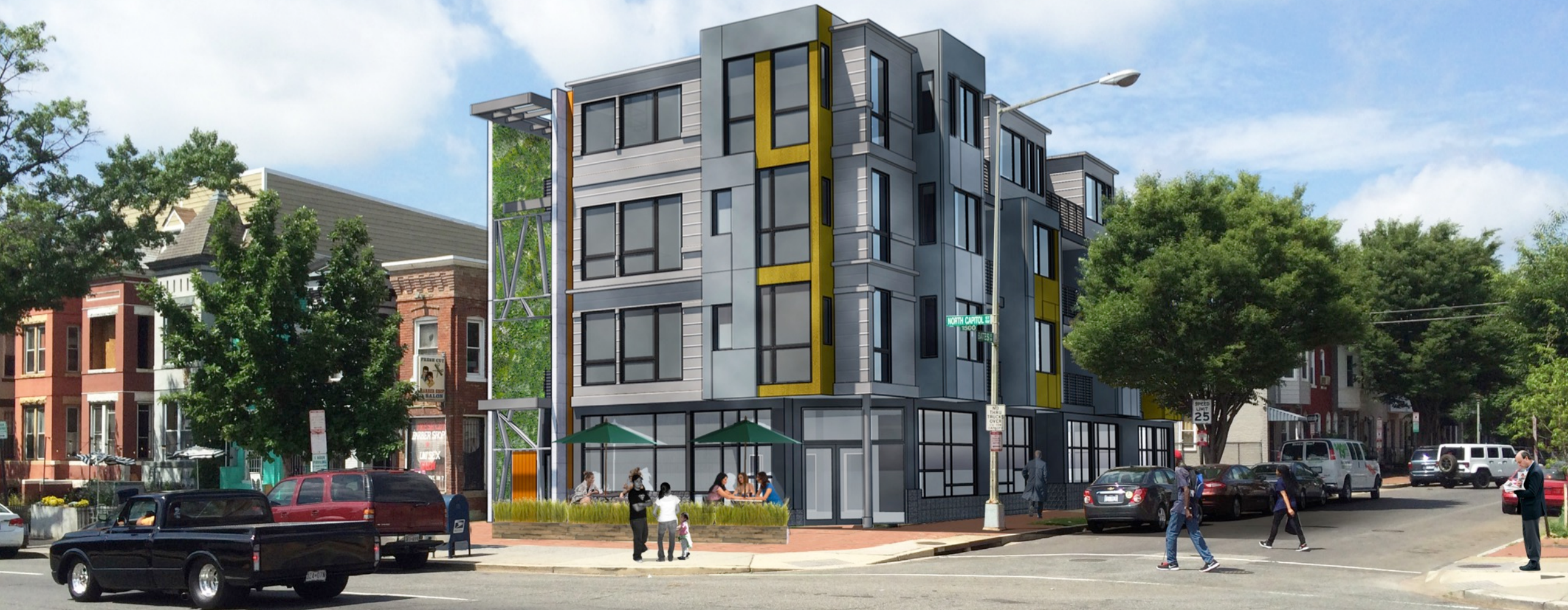
view from North Capitol Street
